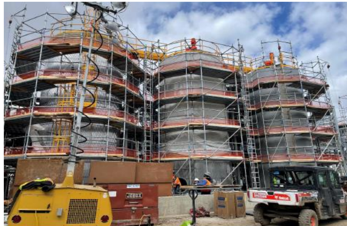
Insulation being applied to new Polymer Modified Asphalt tanks
